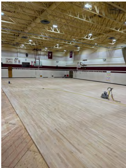
Over the summer our property services staff were busy preparing schools for the return of students. One of these projects was this repair to the gym floor at Islands Consolidated School. The photo on the left shows the floor after sanding, with several boards removed in preparation for replacement. And the photo of the right was taken just before the sealer was applied.
